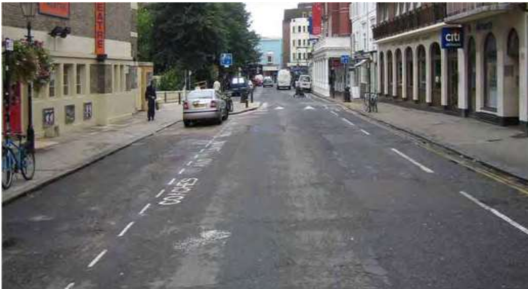
New road, Brighton before renovation. Source: (Living Streets, 2016)
